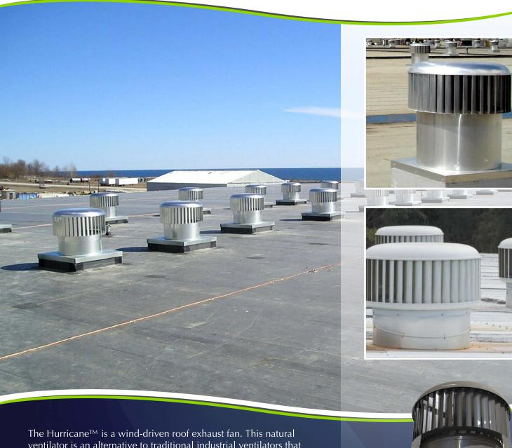
The Hurricane™ is a wind-driven roof exhaust fan. This natural ventilator is an alternative to traditional industrial ventilators that perform poorly and consume energy. Natural ventilation is proven to be effective and keep operating costs down.
